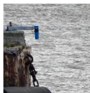
Remote harbor location
